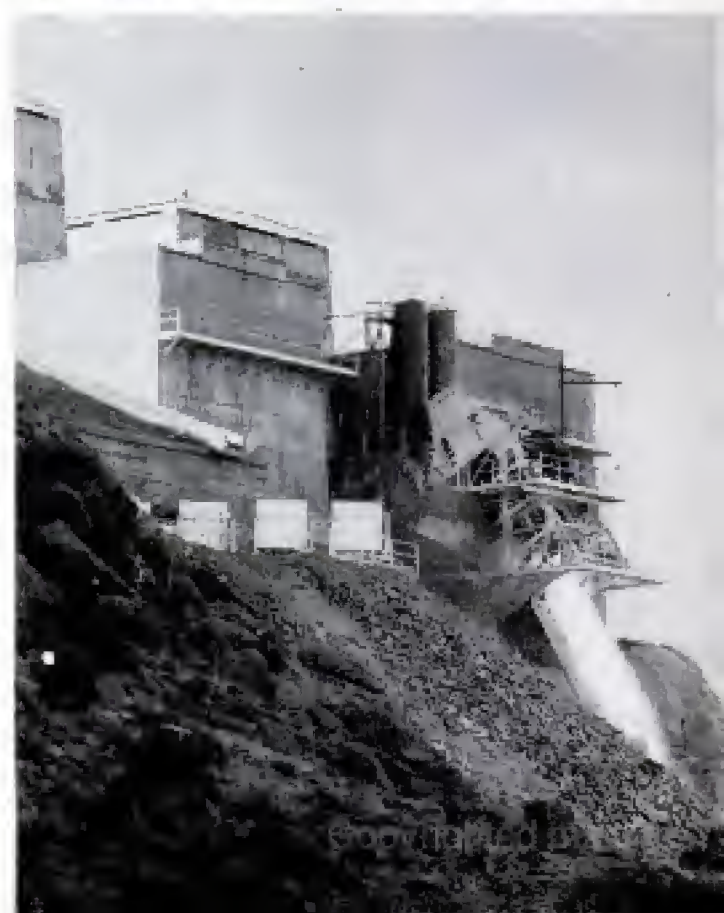
Spillway shown in model at left is designed for the 500,000-pound thrust (below) of a missile in stand
